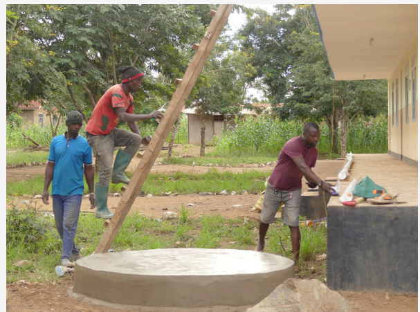
Site 6 — Mbagwi Primary (during construction)
