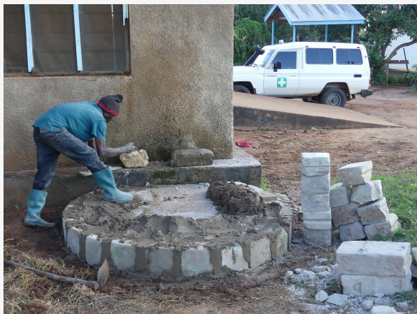
Construction — Concrete Base
